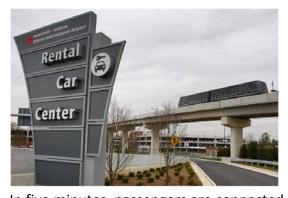
the RCC is an elevated train, called the ATL SkyTrain. In five minutes, passengers are connected from the Airport station at the CPTC to the RCC, the Georgia International Convention Center (GICC), multiple hotels and office buildings. The train operates six dual-car trains which can transport 100 passengers and their baggage.
