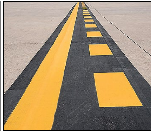
Movement Area Boundary Marking
