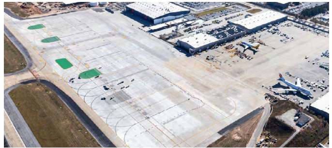
South Deicing Complex completed in 2022
