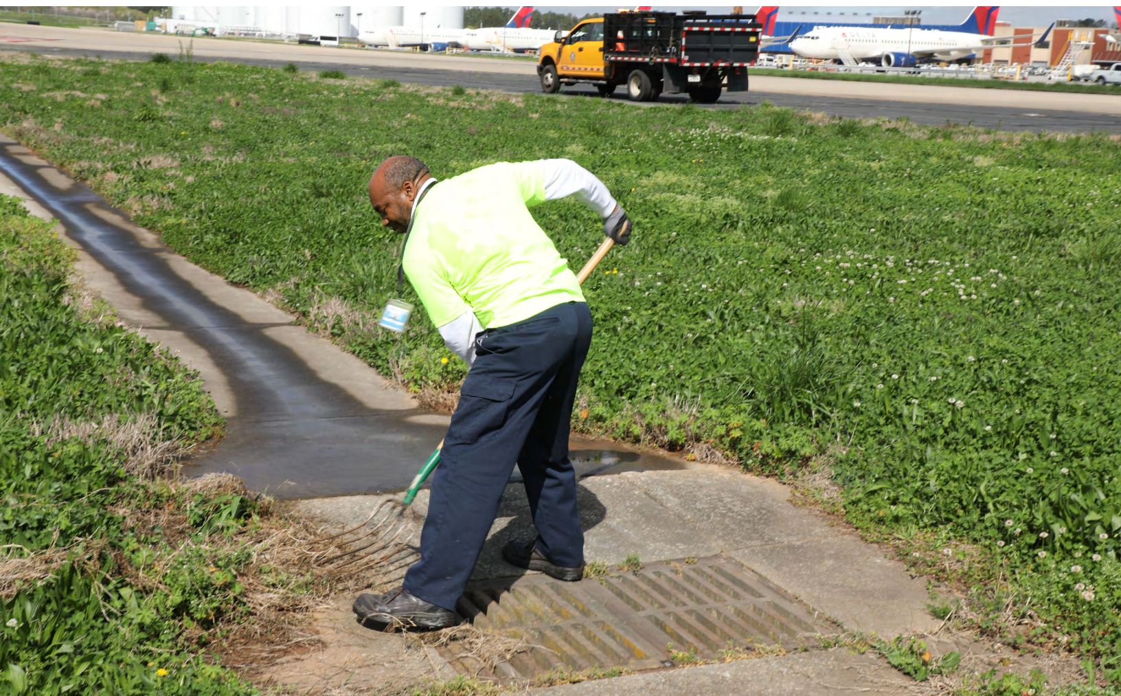
DOA Stormwater Infrastructure preventative maintenance
