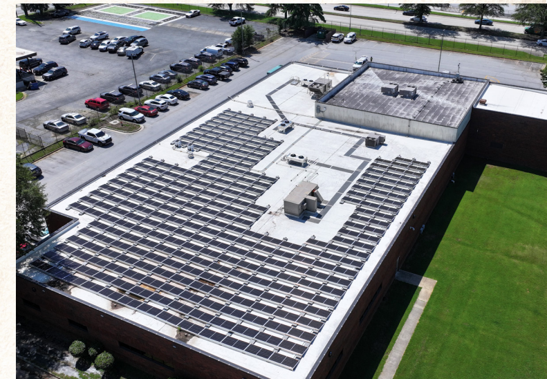
Solar panel installation on roof of C4 building
