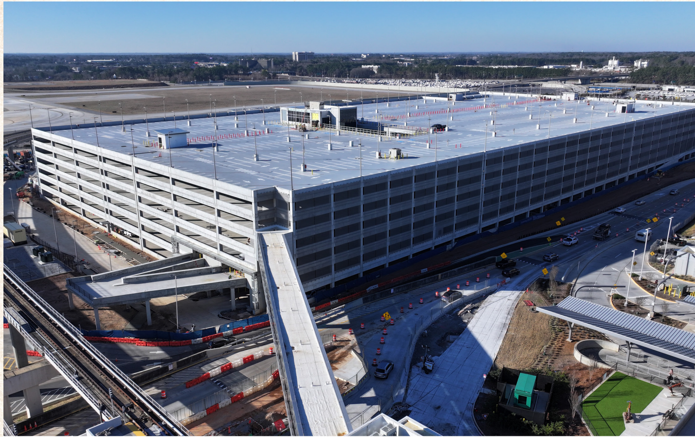
South Red Deck nearing construction completion
