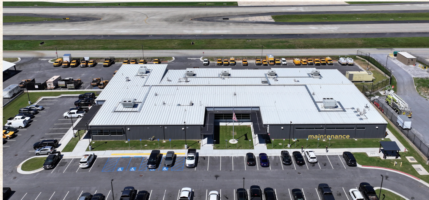
Airfield Maintenance Facilities
