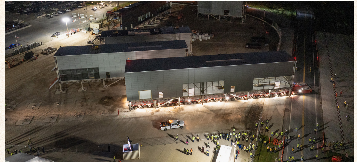
First modular move for the Concourse D Widening project
