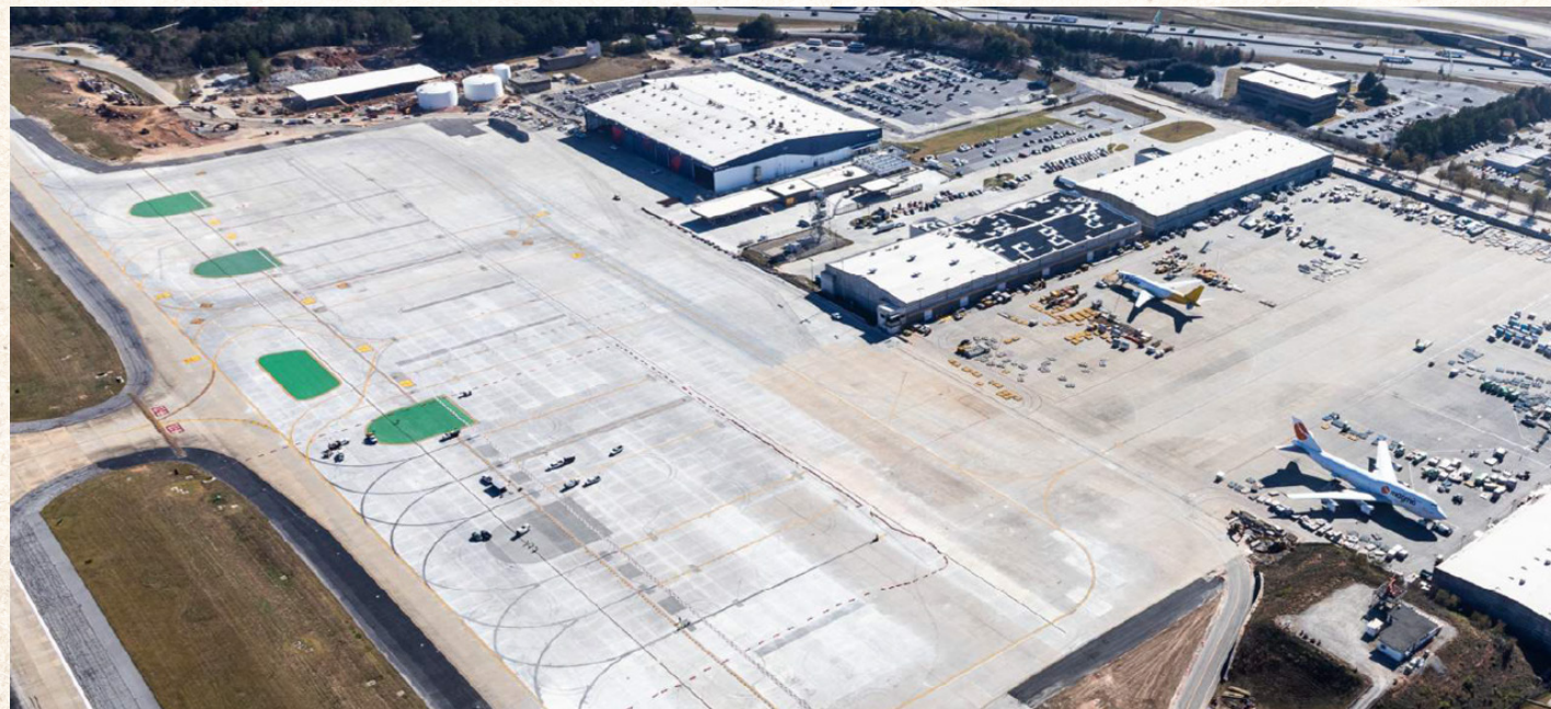
South Deicing Facility
