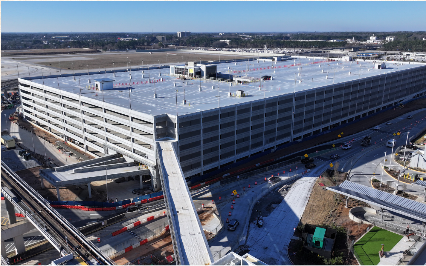
South Red Deck nearing construction completion
